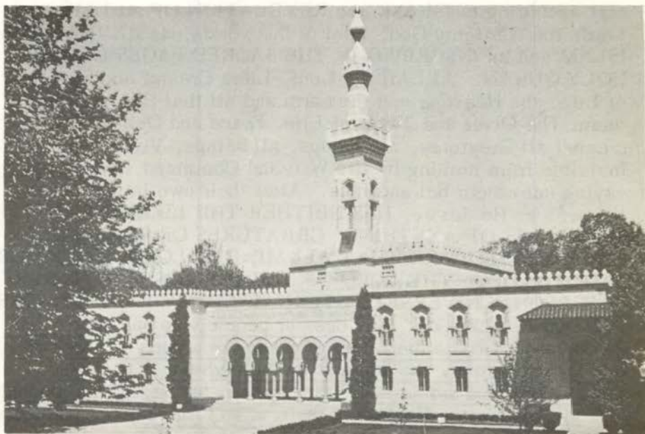
The Washington Mosque. Located at 2551 Massachusetts Avenue, Washington, D. C.
